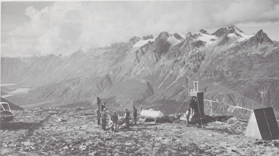
Mountains "scrape the sky" in a breathtaking panorama as FAA technicians put finishing touches on one of three new communications units atop the Lake Clark Pass area.
