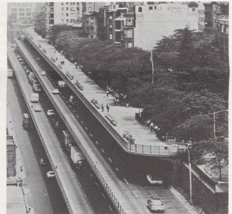
Penetration of the Brooklyn-Queens Connecting Highway required no extra land in addition to the freeway right-of-way for this over-the-highway promenade in Brooklyn. Freeway right-of-way itself is only 50 feet wider than the old street over which the entire modern structure is set.
