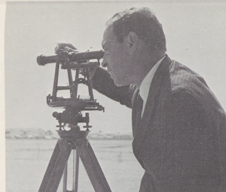
Willis frequently relies on his transit to verify accuracy of elevations during on-site inspections of construction now under way at the new North Perry Airport.
