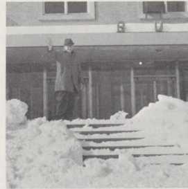
Eastern Region Budget Chief Neil McGroarty waves from front of Federal Building after it was cleared by GSA maintenance personnel. Snow accumulation rose to five feet in front of building as result of high winds and drifting.
