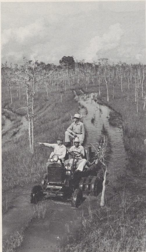
Airport engineers require unusual equipment to get around while building new supersonic airport. Their "swamp buggy" is a converted "Model A" modified to ride high off the ground and above ever-present swamp water. Oversize tires enable the buggy to plow through sticky mud, mire and thick grass covering airport site.
