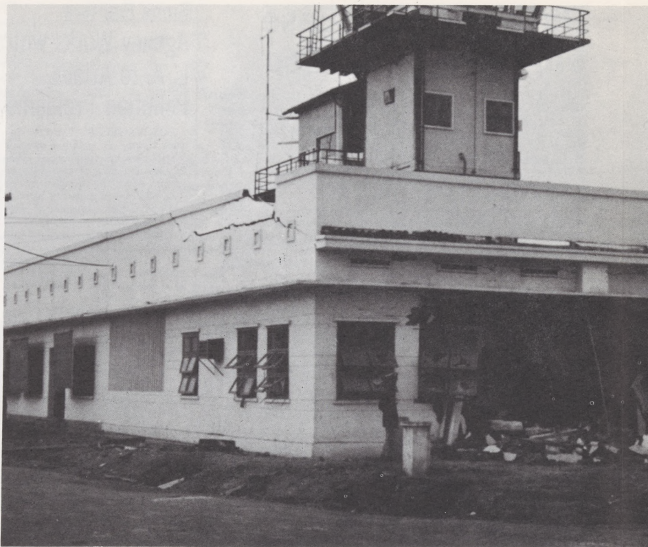
A VC rocket destroys a wall of the CAAG training office at the Tan Son Nhut Airport during the Tet action.
