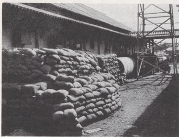
The Saigon Center is now sandbagged even higher and more heavily to guard it from enemy attack. Bunkers also have been constructed nearby as rocket-proof shelters for personnel.
