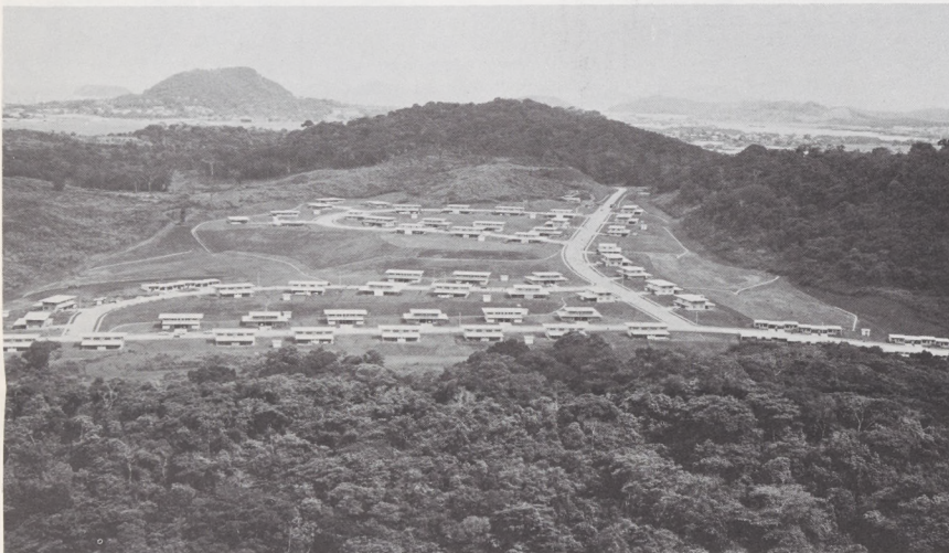
Cardenas Village, a complex of modern split level duplexes, serves as a "home away from home" for many FAA personnel stationed in the Balboa area. Nestled in the tree-studded hills of the Panama Canal Zone, the suburban community thrives in striking contrast to the silent forests peculiar to the vicinity.
