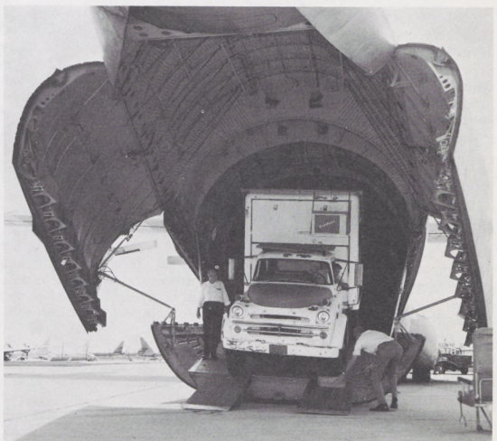
A 16,000-pound portable/mobile VOR test unit of the Southwest Region is loaded aboard an Air Force C-133 transport at Carswell AFB, Fort Worth, for emergency airlift to Wake Island. The unit is substituting on Wake in providing VHF nav aids for aircraft approaches and departures until the permanent facility, which was damaged in Typhoon Sarah, is restored.
