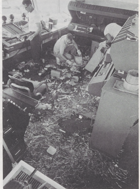
Tower Chief Bob Bailey (left) and crew begin cleanup of the damaged tower cab. Bailey checked the cab after the initial high winds passed over Wake and found it had survived. But 160-mile winds that followed the lull of the typhoon eye blew in all the windows and extensively damaged the equipment inside.
