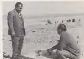
CENTO specialist examines radar tower foundation.
