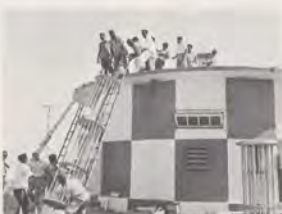
Technicians hoist antenna on VOR in Pakistan.
