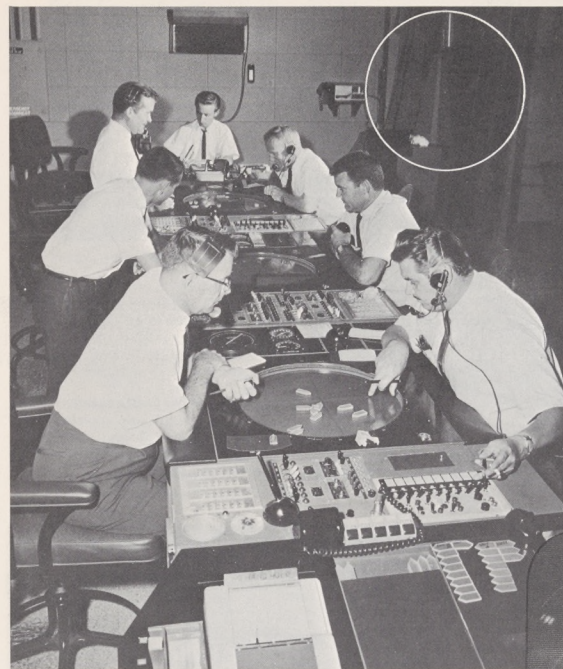
The television set-up for Honolulu's improvised "bright display" system is shown from both ends. At left in the TRACON room the television is circled. Below is a close-up of the TV screen at the "local" position in the tower. A prototype of the system being procured by FAA is being tested in Atlanta.
