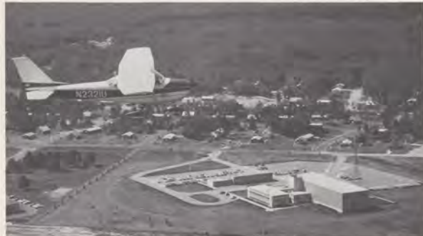
The Boston Center at Nashua, N.H., controls general aviation traffic as well as the huge jets which fly the transoceanic routes. Here a Center Flying Club aircraft flies over the facility which is nestled in a magnificent forest area.
