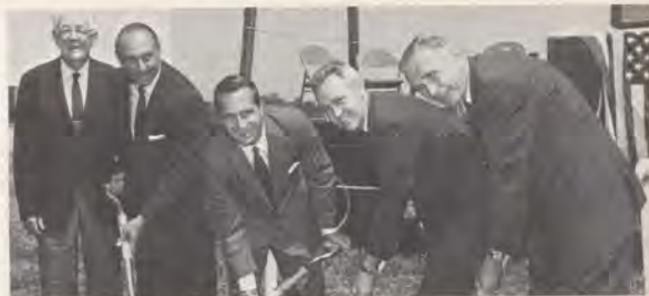
A battery of ground breakers marked the start of construction of a new control tower at the Westchester County Airport, White Plains, N. Y. Breaking the ground were, from left, James Harding, County Public Works Commissioner Edwin Michaelian, Congressman Ogden Reid, FAA's Eastern Region Director Oscar Bakke and Westchester County Airport manager John L. Remmert.
