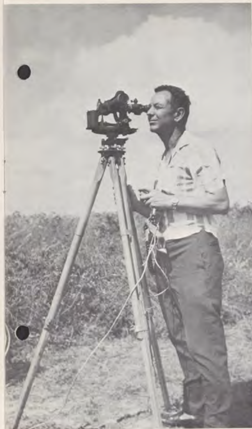
Maurice McGranahan of the Miami Area Office takes a sighting through a theodolite during a VOR site evaluation check at Santa Cruz, Bolivia.
