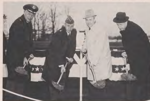
Top brass dig in at March 4 ground breaking ceremony for a new FAA tower at Andrews Air Force Base. From left are: Brig. Gen. John S. Chandler, Commander of Andrews; Major General Rollen H. Anthis, Commander of the Headquarters Command; Oscar Bakke, Eastern Region Director, and Stanley W. Henceroth, Washington Area Manager.
