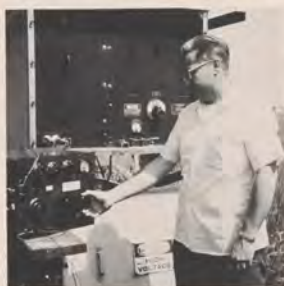
Technician Robert Haen of the Buffalo, N. Y., Airway Facilities Sector uses Z Box Number One which is used to check low frequency nav aids still in the airway system.
