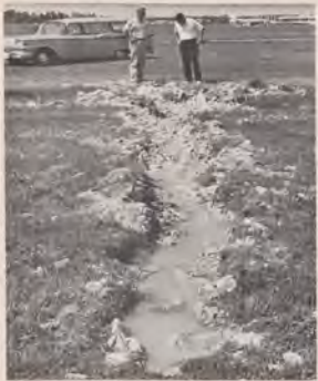
Lightning struck at Columbia, S. C., Metropolitan Airport, hitting the tower and the field where it left a trench 45 feet long. William A. Davenport and Marvin T. Love check the damage.
