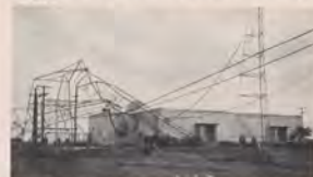
Several towers "hit the dirt" and others were damaged when high winds whistled through Dyess AFB RAPCON.
