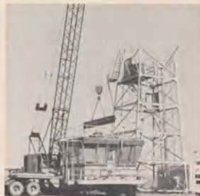
Like dismantling an erector set, the 15-year-old McCarran Field Tower, Las Vegas, comes apart piece by piece for its road trip to Thunderbird Field, six miles away.
