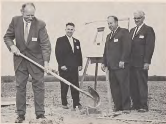
Allan E. Horning, chief, Western Region Airway Facilities Division, breaks ground for a new air traffic control tower at Hillsboro, Ore., while city officials, from left: John Crockett, Emery Dye and J. W. Barney, await their turn.
