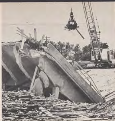
A bridge was washed out by floods.
