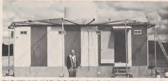
Once the mobile nav aids are at the site, the wheels are taken off and the body is mounted on concrete pillars.
