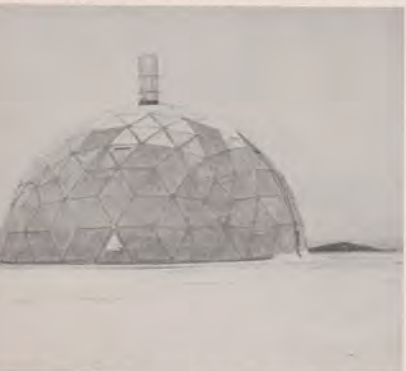
Above: New 55-foot-diameter geodesic fiber glass dome encloses the conventional VOR antennas at Mullan Pass. Before installation accumulated snow affected VOR's accuracy. Below: Inside dome, normal antenna enclosure is at far right. Ample space is provided inside for electronic checks and measurements.
