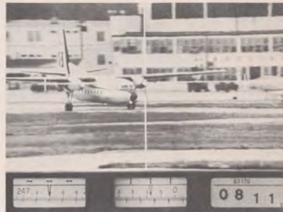
Below: Even if cross-hairs of theodolite sight are not precisely aligned on the predetermined bulls-eye of the target, data processing operators can make corrections using movable cross-hairs which compensate for the error. The theodolite facilities at NAFEC are available to industry on a rental basis.
