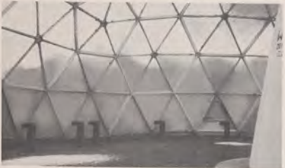
Above: New 55-foot-diameter geodesic fiber glass dome encloses the conventional VOR antennas at Mullan Pass. Before installation accumulated snow affected VOR's accuracy. Below: Inside dome, normal antenna enclosure is at far right. Ample space is provided inside for electronic checks and measurements.
