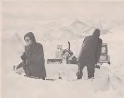
Mullan Pass Systems Maintenance Service electronic maintenance technicians Russell L. Miller (left) and Fred E. Manthey clear the theodolite pedestal prior to a flight check. Storm blew door off shelter and the interior filled with snow.
