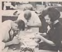
Above: Umpires-for a defense readiness exercise check proficiency in use of Geiger counters. A radioactive substance was found under the paper cup in foreground. Left: Dosimeters which will show the cumulative radiation exposure of the wearer are being charged prior to being issued during an exercise. They are available for all employees for exercise or emergency use. Right: Washington FAAers return to their desks following all-clear. Such civil defense exercises are part, but far from all, of the readiness program.
