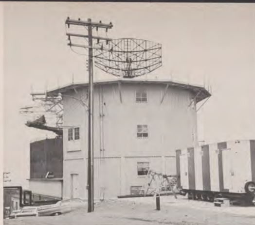
Above: MERF-1 on location at Bucks Harbor, Maine. Trailers for all FAA mobile facilities are very similar in outward appearance. Inside, however, they are designed to support or replace a variety of specific facilities. MERF-1 is a complete air route radar surveillance transmitting and receiving system which is temporarily providing FAA radar service in the northeastern part of the United States. Right: Lester Smith, Eastern Region electronic technician, replaces chassis in the video distribution cabinet. MERF-1 designers provided room for an operating area and an equipment working area.
