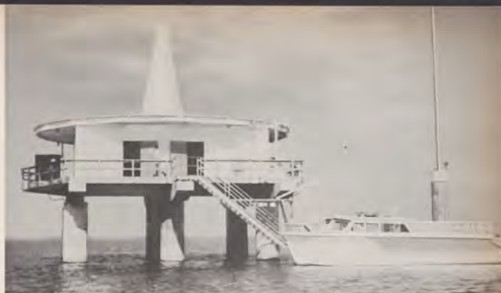
There's nothing wet about this VORTAC's signal even though it's four miles from the shores of Lake Ponchartrain. New Orleans SMS technicians regularly ride the 38-foot launch to service its complex of electronic equipment.
