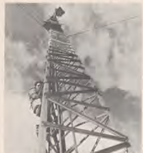
High places are not new to Walter Christiansen, but the former paratrooper would find a parachute cumbersome in his present job as an FAA electrical lineman.
