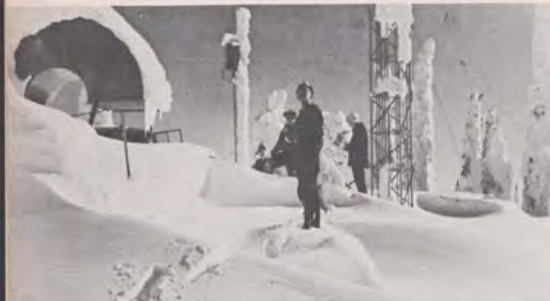
Snow-covered RCAG building on 6,700' Big Mountain near Whitefish, Mont.
