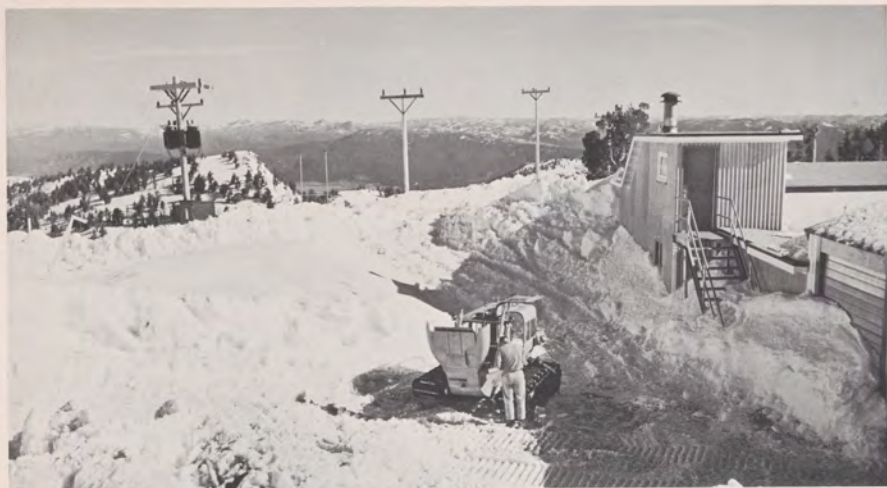
The picture tells the story. Maintenance technicians get through in Sno-cat and the facilities stay on the air.
