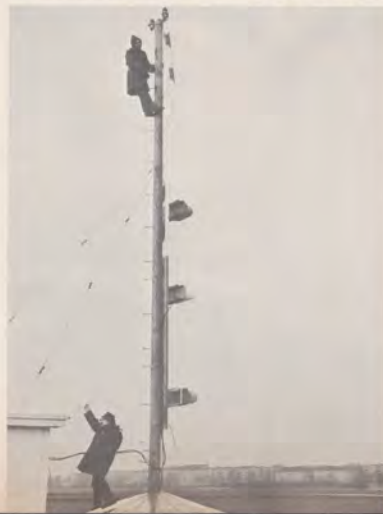
Above: typical post-war German apartment houses surrounding Tempelhof Airport. Localizer for runway 27L is in foreground. Below: technicians of the Berlin Aeronautical Unit install some of the monitoring equipment on the mast of the capture effect glide slope antenna. Rain-streaked roof of hut gives a clue to the kind of weather prevailing a large part of the year.
