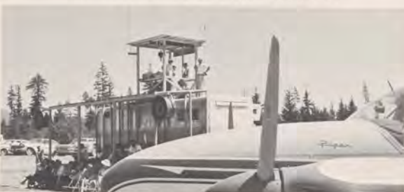
At Prospect, Ore., FAA provided a temporary tower for airport dedication and flight. Field was built largely through local contributions; tower, provided by Medford CS/T. Richard T. Smith, Medford facility chief and Gilbert J. Thiel, Medford controller, manned tower. Robert E. Barnum, SMS-430, provided technical support.
