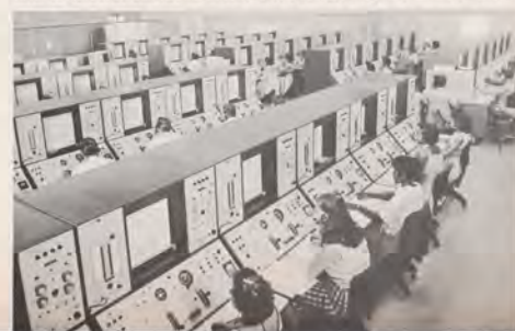
These 60 generators comprise the aircraft input of NAFEC's large ATC simulation system.
