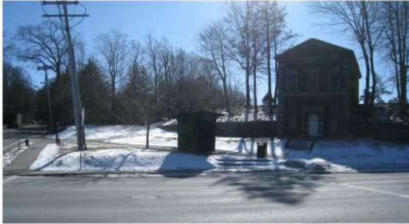
View of the Reservoir Gatehouse (with temporary shed)
