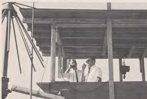
Typical of the special services provided by FAA for the women flying in the recent All Women's Transcontinental Air Race, popularly known as the "Powder Puff Derby," was this temporary control tower at Cape Girardeau, Mo. Erected by the local airport officials, it was staffed by controllers from the Lambert-St. Louis Tower. On duty in the open-air cab are, from left: Paul Marchbanks and Gil Wallace, Jr. After race ended contestants rounded up at NAFEC for the third time.
