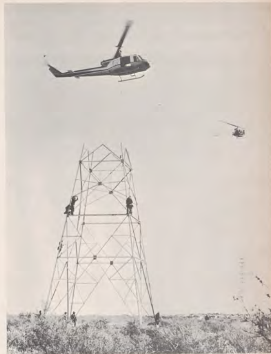
Supplies are moved quickly to remote area by helicopter using external slingload. 'Copter's accurate placement (right) of sections helps build tower in 30 minutes.
