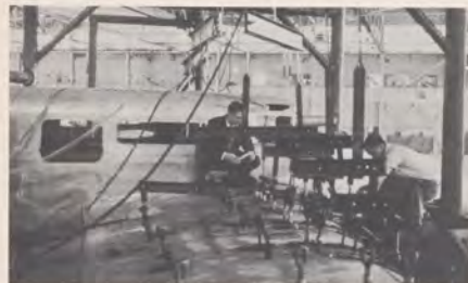
Calvin L. Stoner inspects "whiffletree" before loading wing with about 24,000 pounds. Below: 7,000 pounds of lead are laid on stabilizer to determine its failure point.
