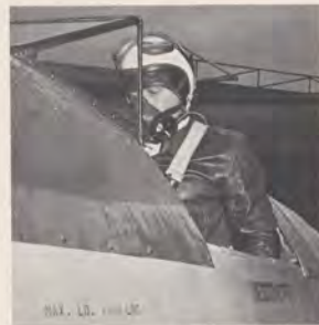
(Above) The Well dressed ag pilot about to perform his chores not so high above a cultivated field, is toggled out in "hard hat", safety harness, and respirator. Open cockpit flying brings the pilot into proximity of the poisons he sprays. (Right) "Copter dusting" accounts for two per cent of dusting in the Southwest Region. Initial cost of equipment is high.
