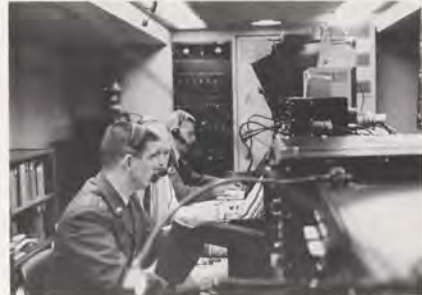
Lt. C. H. Anderson, foreground, mans the surveillance scope while E. J. Formiller (center) handles incoming flight data. AIC R. H. Hinton conducts a precision approach for an incoming jet fighter of the Air National Guard based at Duluth.
