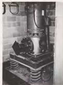
Loss of this handsome building (top) in an atomic attack would not destroy vital communications buried deep under its foundations. Shock-mounted pump (r.) gets water from wells in underground facility. In meeting at the Center (below, r.) are: (l. to r.) J. W. Skolaut, FAA Asst. Readiness Officer; E. A. Addington, FAA Defense Readiness Officer; Mrs. Z. Whatley; W. Parker, OCD Regional Director; L. T. Holland, Asst. Dir.; G. Hastings, Regional Dir., OEP; and V. Twaddell, OCD Field Service Dir. Defense Center building "going down" during construction of heavily-reinforced concrete walls up to 42 in. thick.
