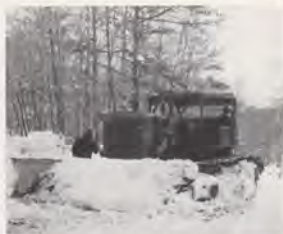
Bulldozer blade makes a "clean sweep, fore and aft."
