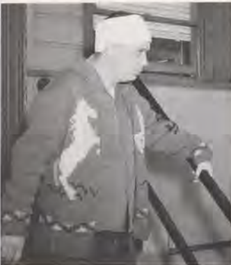
Robert L. Daymude escaped with minor injuries when the Anchorage tower collapsed.
