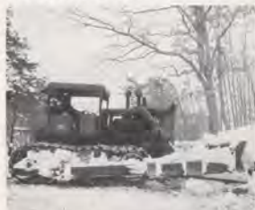
A bulldozer opens access road to Ravine, Pa., VORTAC.
