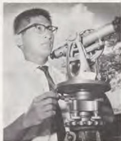
Ed Masuoka, Facilities Engineer, operates a transit to find airport approach obstructions.
