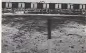
The new antenna array of Directional Waveguide ILS Localizer at the Greater
