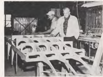
Burrell Tibbs, veteran pilot and retired employee of Boeing Aircraft, inspects the hull of the replica of the Benoist Airboat. Tibbs helped to build the first airboat 50 years ago. Working on the aircraft is Louis Hoss, owner of the H&H Cabinet Shop.
