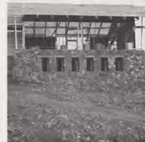
This is the radar site on Brushy Mountain where crew quarters were built. Partially completed quarters show natural stone used to blend quarters with the terrain.
