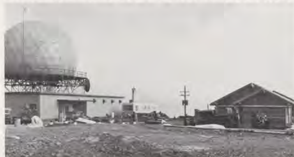
This is the radar site on Brushy Mountain where crew quarters were built. Partially completed quarters show natural stone used to blend quarters with the terrain.
