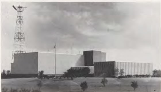
FAA Air Route Traffic Control Center buildings are the culmination of years of planning and experience and are designed to accommodate all known aids and devices for air traffic control, with the further feature of being expandable to house future developments. The tri-level structures, functional and contemporary in design, are built of steel and concrete, and have approximately 54,000 square feet of floor space, featuring an 11,000-square-foot control room.
