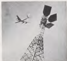
Microwave towers are used to bring radar information from the antenna sites to Air Route Traffic Control on scopes.
