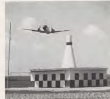
The VORTAC, which gives pilots both direction and distance information, is the FAA's modern aid to air navigation.
