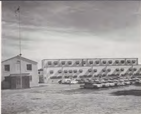
Building 1 and 2 at Southwest Regional headquarters as visitors see them from the main gate.
