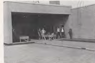
The 'copter enables the newspaper to cover a nine-county area where some 350,000 people reside. (Below) The rails on which the landing pad moves in and out of the rooftop hangar are clearly visible in this view. 'Copter can be moved and ready to fly in minutes.
