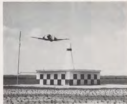
(Left). This old sentinel of the airways—the Low Frequency Radio Range at Florence, S. C.—is the last of the "old timers" in the Southern Region to be decommissioned. They are being replaced by the modern Very High Frequency Omni-directional Radio Range with TACAN at right. New installation is more efficient.
