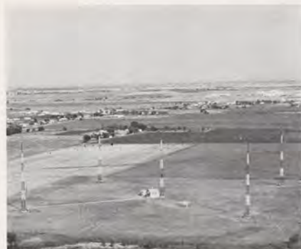
(Left). This old sentinel of the airways—the Low Frequency Radio Range at Florence, S. C.—is the last of the "old timers" in the Southern Region to be decommissioned. They are being replaced by the modern Very High Frequency Omni-directional Radio Range with TACAN at right. New installation is more efficient.
