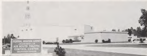
Center Area Manager Headquarters at Jacksonville is in the Jacksonville ARTCC Building. From this place, a unified air traffic, systems maintenance, and supply team under an Area Manager create a common FAA system.
