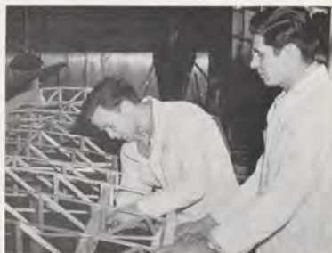
Paul Koppin (left), who escaped from East Germany and came to Alaska as an immigrant, works on a wing brace under the supervision of Joseph Fitzgerald of Gills Aircraft Service in Anchorage, Alaska. Eighteen months of supervised work or successful completion of an FAA approved school are prerequisites for becoming certified as a mechanic.
