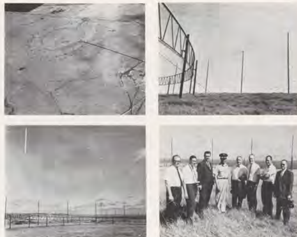
Top, left: Luneburg Lens receiving antenna at Molokai. From this angle (top, r.), the antenna looks like a circus safety net. Grid pattern (below, l.) of antenna can concentrate many waves from many directions and frequencies simultaneously. Inspecting the installation are: H. O. Williams, Area Coordinator; J. Libbert, NSA; R. Gale, PC Director; Gen. G. A. Blake, USAF; L. Rosen, NSA; Dr. R. Tanner, C. Rose, Project Superintendent for the lens on Molokai; and W. A. Gaspar, Chief, Compliance and Security, PC.
