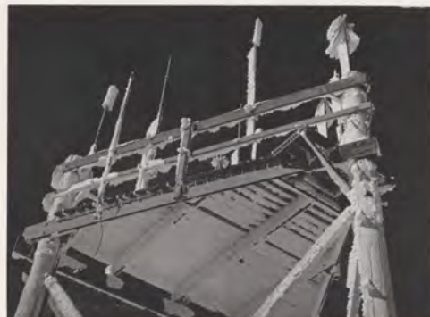
Ice on Sandia Mountain antennas is problem for personnel in Albuquerque's SMS 102.
