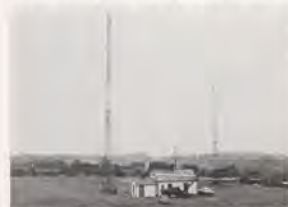
Low frequency towers stand erect (left) after 27 years of uninterrupted service in the Pittsburgh area.
