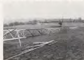
Demolished tower structures mark end of low frequency facility in Pittsburgh after 27 years' service.
