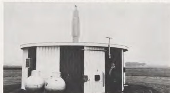
State-owned VOR's come in assorted shapes and sizes but all do the job they were intended to do, provide safe, economical radio navigational assistance to pilots in remote areas not served by Federally-owned facilities. Above is the Mankato, Minn., VOR which has services remoted to Minneapolis Flight Service Station.
