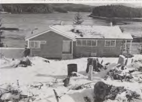
Quarters building at recently decommissioned Angoon Repeater Station.
