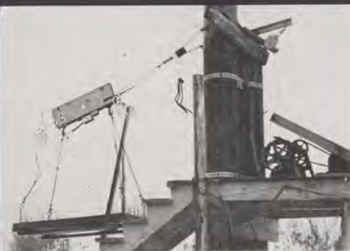
Tramway runs from engine house near shore to housing at Sunset Cove.
