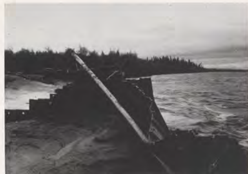
Concrete dike at Galena damaged by water and ice chunks 25 feet wide and 40 feet thick. Below, aerial view of VORTAC and site undermined by flood as new channel eliminates roadbed.
