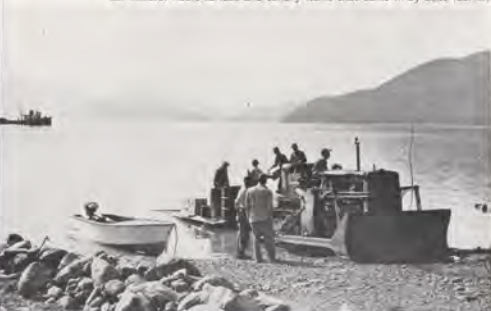
Supplying Rodgers Point was a problem in logistics. A marine railway car (above) hauls various and sundry items that came in by boat (below).
