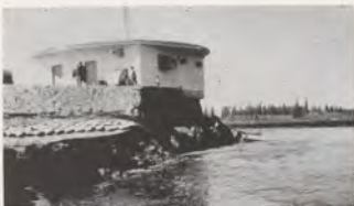
VOR at Fort Yukon undermined by the flooding of the Yukon and Kuskokwim. Village is at the confluence of four rivers.
