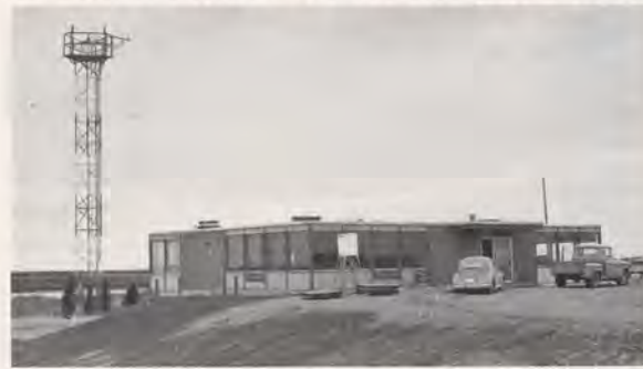
New King Salmon FSS building houses numerous facilities.
