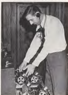
Voice recorders are not new in ATC operations but modernized equipment marks the change from the old Edison recorders (left) to bank of 22 channel, 16-hour tape recorders on one console on page 5.
