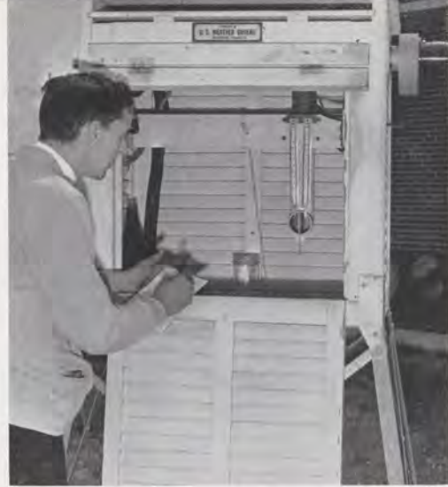
Boozer waits for fan (located above thermometers) to circulate air around the two instruments before taking hourly reading. At night a "Clinometer" is used to compute ceiling.
