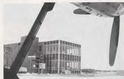
An outside view of the Mason City Flight Service Station.
