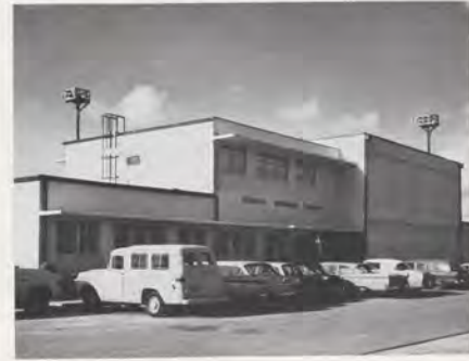
The new Guam International Flight Service Station (IFSS) Building, commissioned and dedicated last May, where 175 employees and their families took refuge from Karen and where Joe Price temporarily housed radio equipment.
