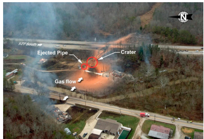
Figure 2.10 Exploded Buried Pipeline Sissonville, West Virginia (Source: NTSB, 2014).
