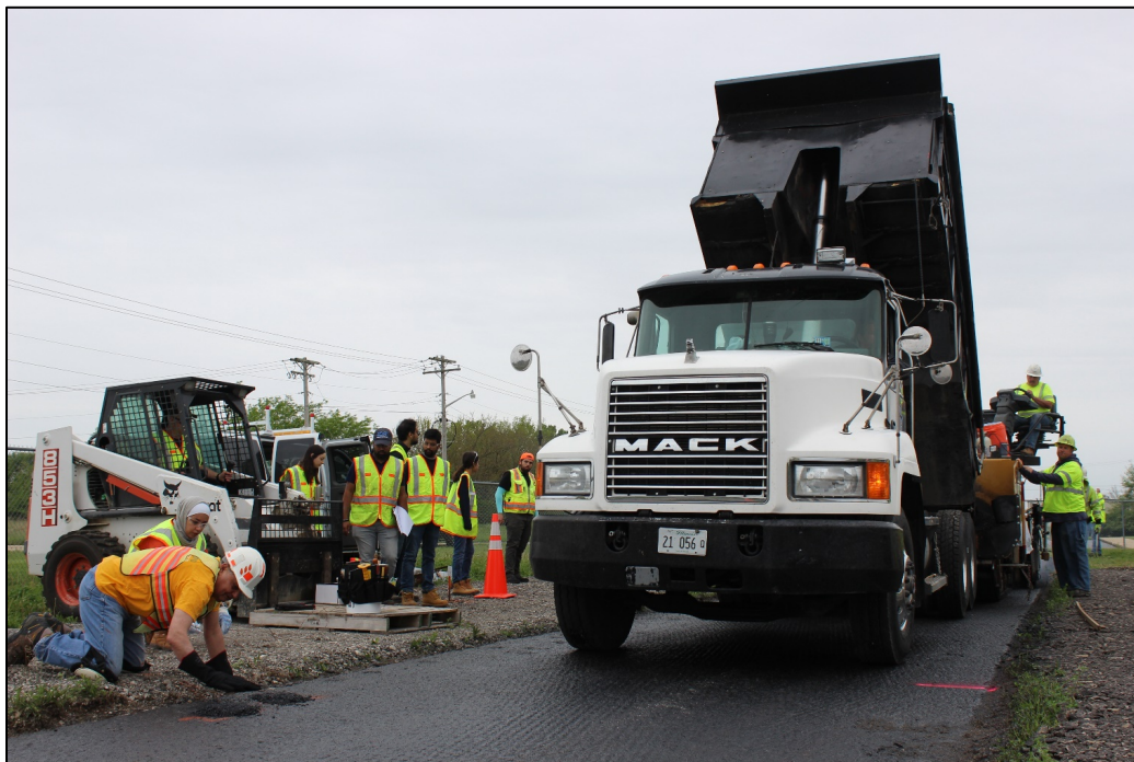
Figure 55. Photo. Thermocouple placement before paver.
