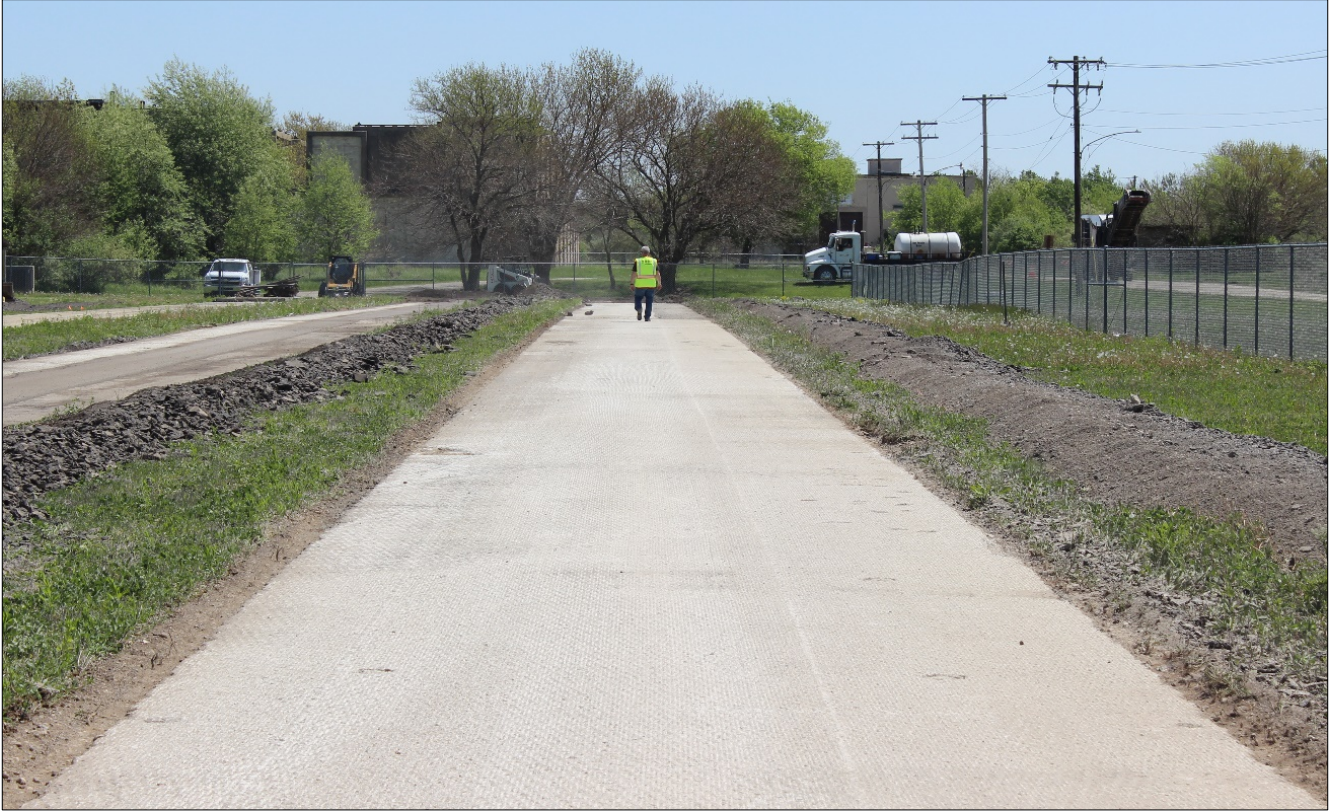
Figure 21. Photo. Bare CRCP supports the HMA and SMA layers.
