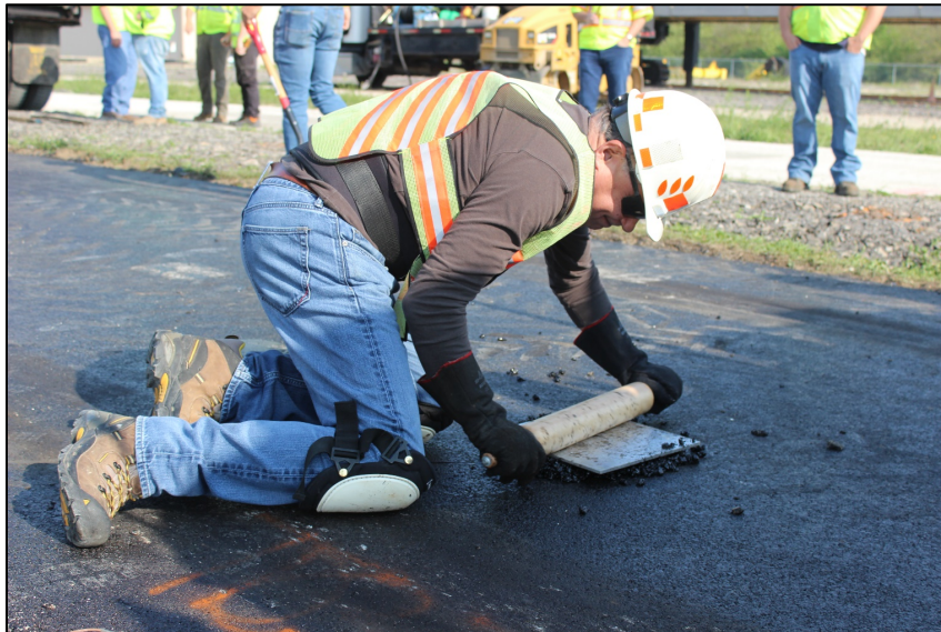
Figure 53. Photo. SMA compaction over a strain gauge prior to paving.
