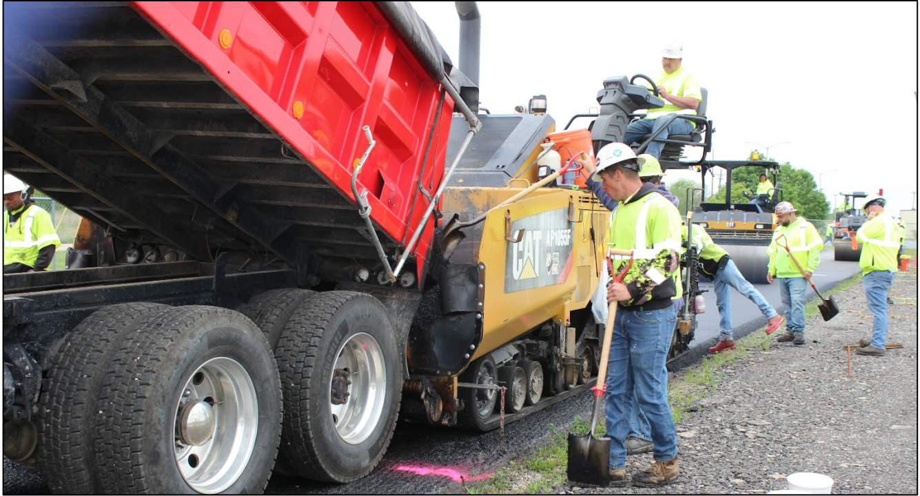
Figure 23. Photo. N90E mix paving.
