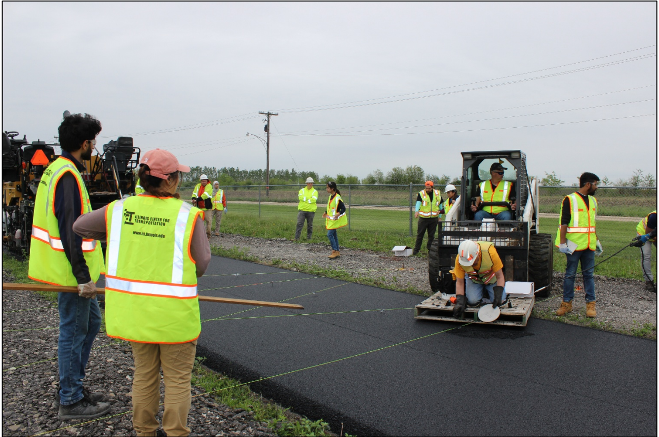
Figure 45. Photo. String and flag instrument location.
