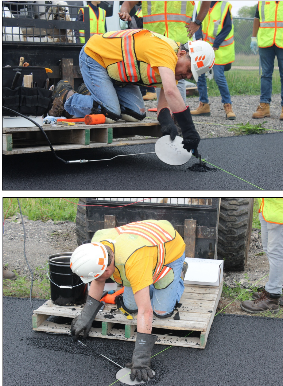
Figure 48. Photo. Placement of a pressure cell on HMA mat before compaction.
