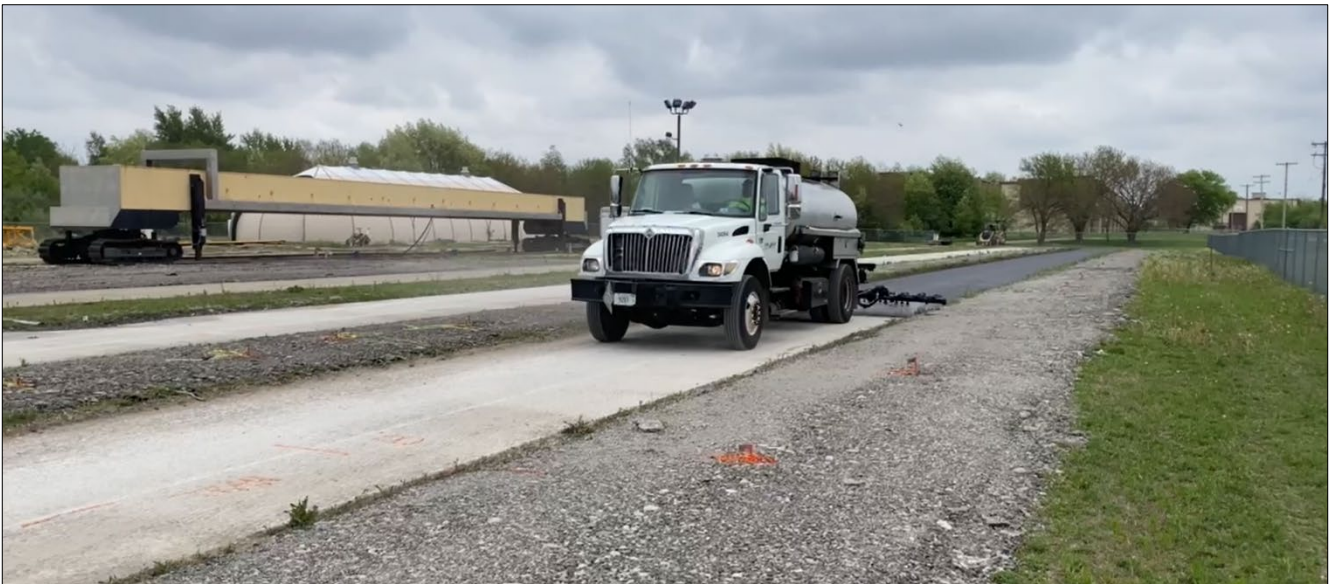
Figure 22. Photo. CRCP tack coat application.
