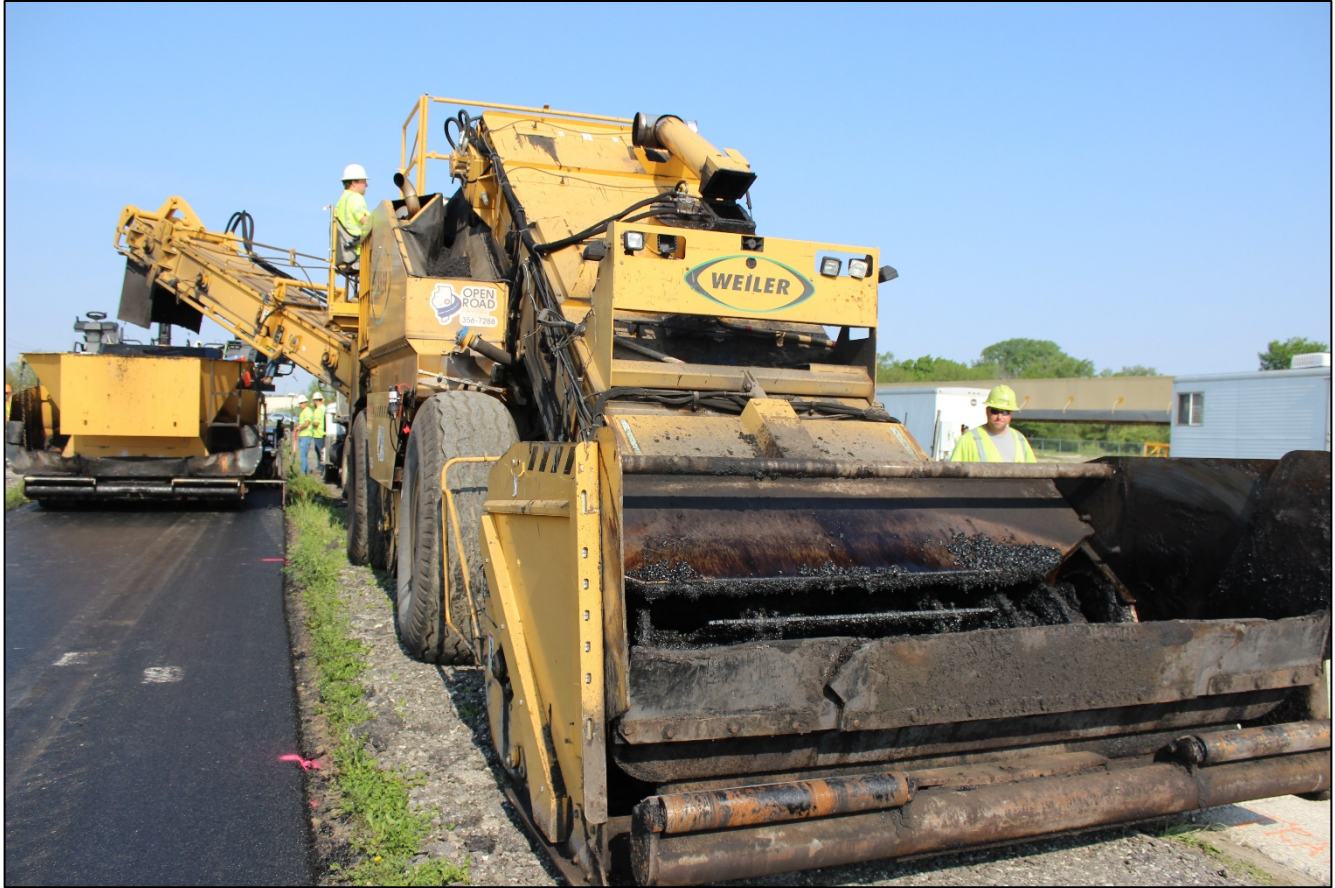
Figure 25. Photo. Material transfer device and paver used to pave SMA sections.
