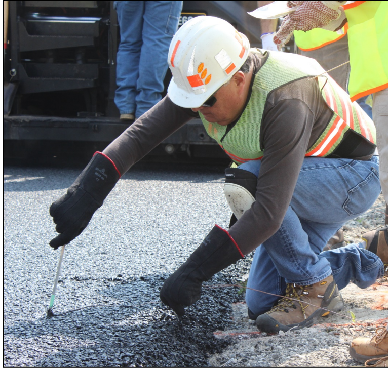
Figure 56. Photo. Thermocouple placement after paver and before compaction.
