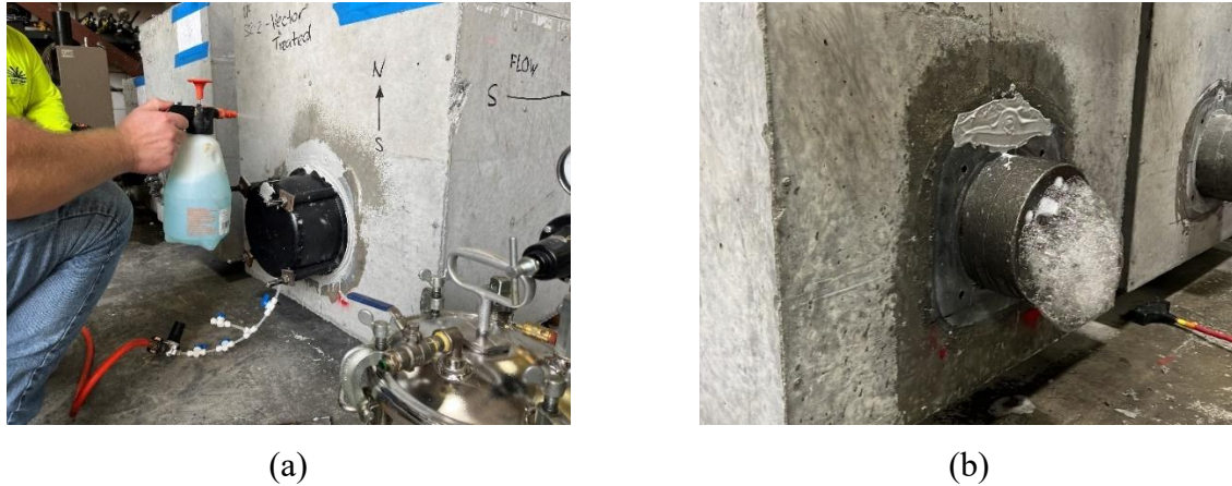
Figure 8.4. Air flow tests on S12-P-T beam: (a) Checking for leaks at the bearing plate-concrete joint at PT live end; (b) Bubbles confirming air flow at the PT dead end.
