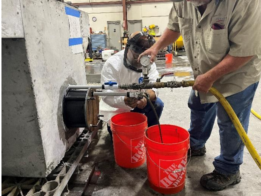
Figure 6.16. Grout injection at PT live end of beam S19-M-U
