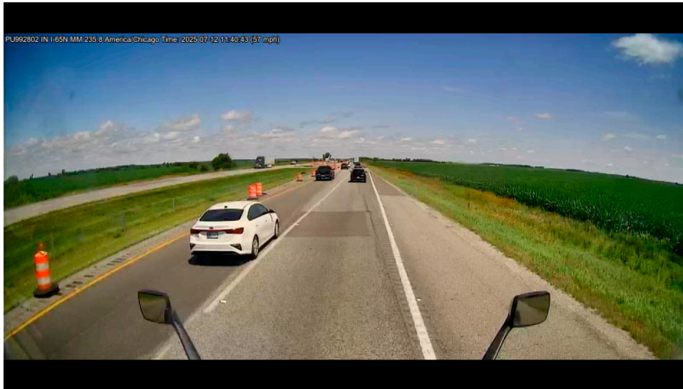
Figure 5.4 Dash Camera Image Along Northbound I-65 Near MM 236 on July 12, 2025, Showing a Double Lane Shift Within a Work Zone.
