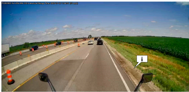
Figure 2.6 Image Showing Inconsistent Right Edge Line Pavement Markings and Inconsistent Lane Widths.
