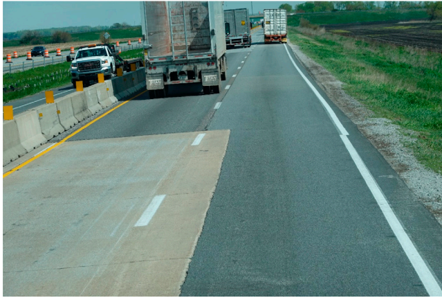
Figure 2.6 Image Showing Inconsistent Right Edge Line Pavement Markings and Inconsistent Lane Widths.
