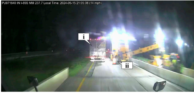
Figure 2.2 Dash Camera Image Showing a Semitruck Driving on the Shoulder Through a Work Zone During a Material Transfer Operation.
