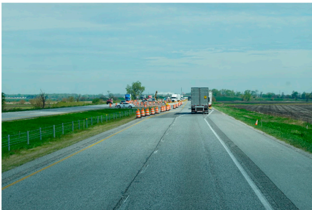
Figure 2.3 A Double Lane Shift Inside of a Work Zone.
