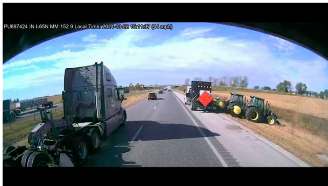
Figure 2.22 Dash Camera Image Showing a Semitruck Traveling by a Work Convoy on the Outside Shoulder.
