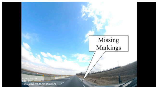
Figure 2.5 Dash Camera Image Showing Right No Right Edge Line Pavement Markings.
