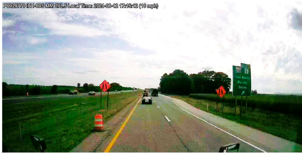
(b) "LANE ENDS MERGE LEFT" Sign 1,000 ft in Advance of Merge Point
