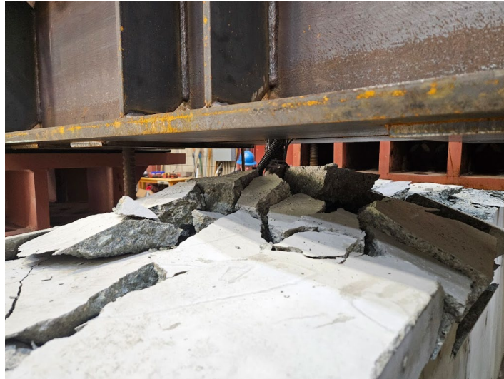
(a) Cracking at the top of the beam
