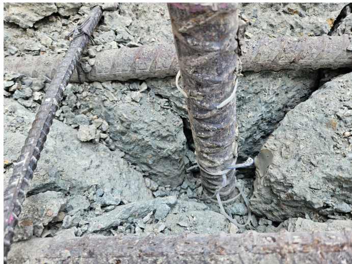
(b) After removing cracked concrete pieces at the top
