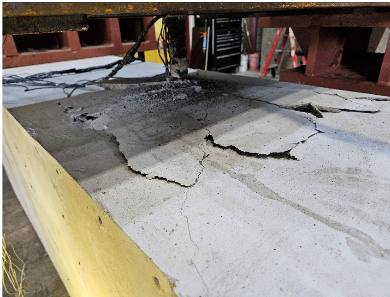
Figure 4.7: Cracking at the top of the beam in Specimen 2
