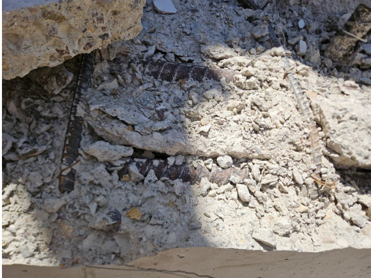
(c) After removing cracked concrete pieces at the top
