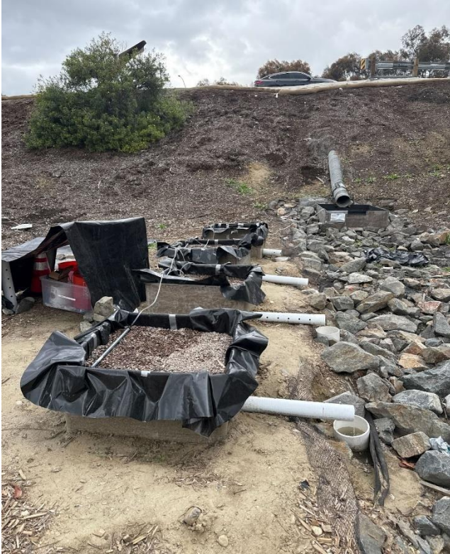
Figure 14.6 Pilot scale experimental setup of the stormwater filtration units.
