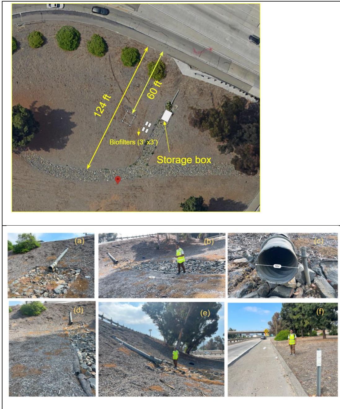
Figure 13.4 Field site 1, inspection for pilot system installation.
