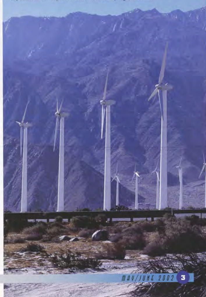
Heat is not the only danger in the desert. These wind generators guard an important mountain pass northwest of Palm Springs, California.
