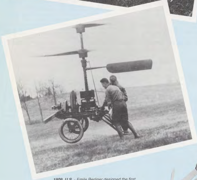
1909, U.S. - Emile Berliner designed the first light-weight radial engine for airplanes and dreamed of "aeromobiles" that would go straight up. Shown is Model A, an unstable design which did get several feet of the ground. He and his son, Henry, would redesign and improve their working model until they finally achieved the first controlled helicopter flight in aviation history in 1924. Model H is also shown.
