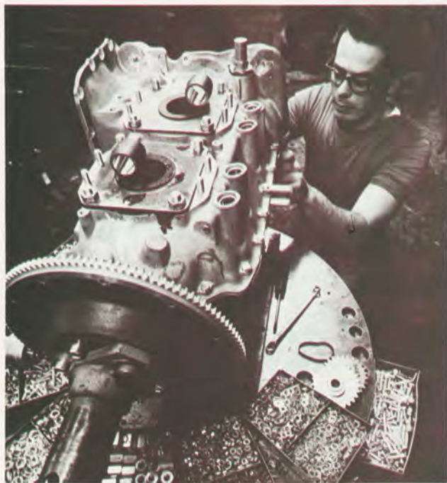
The sum of the parts is many when it comes to airplane engines. Some have over 1,000 individual pieces. Engine at left is a four-cylinder Lycoming, disassembled and cleaned for inspection and replacement of all worn parts.
